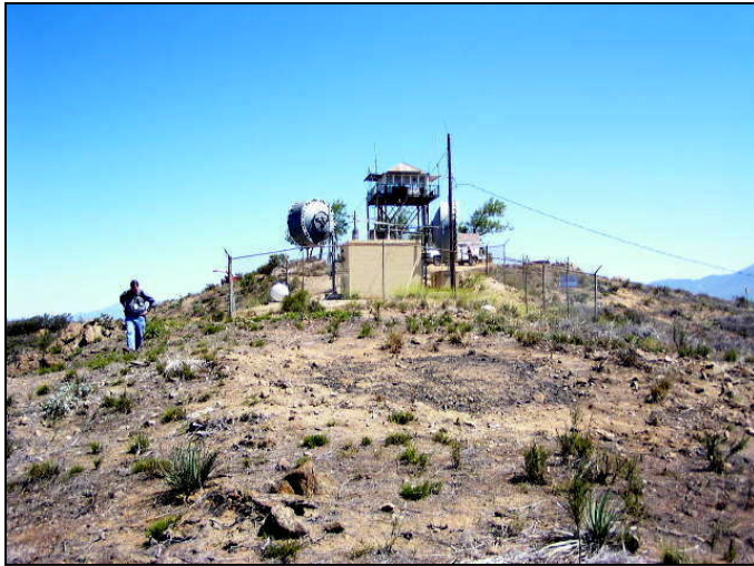
Photograph 3: Overview of Red Mountain candidate location, facing north.
